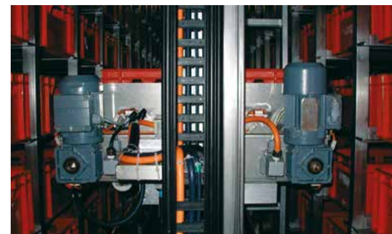
Control cable Chainflex® CF10 in storage and retrieval units for high-bay warehouses. E-chain®: System E2 medium
